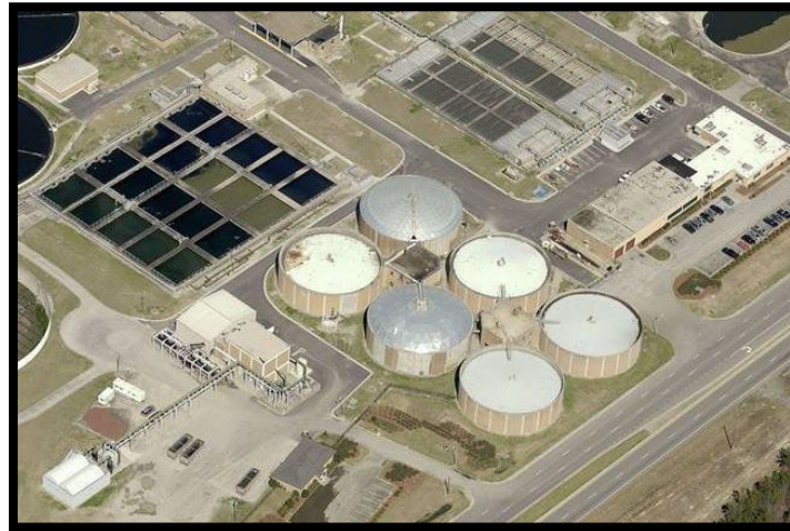
Figure 2: The J. B. Messerly Water Pollution Control Plant
