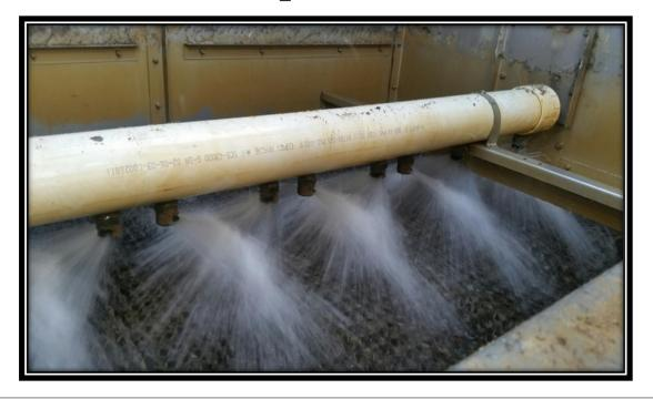
Due to equipment malfunction, the cooling tower's conductivity meter read 14,000 µS, which was 6 times too high. Airman Payne repaired the damaged system and reset the controller back to the normal operational parameters of 2,300  $\mu$ S. No significant hard scale or bio buildup was observed on the nozzles or infrastructure.
