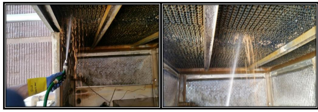
Instead of the hard scale that typically accumulates inside the cooling tower, loose brown mud-like material was found. A garden hose was used to easily remove the mud-like substance from the fill material and the drift eliminators.
